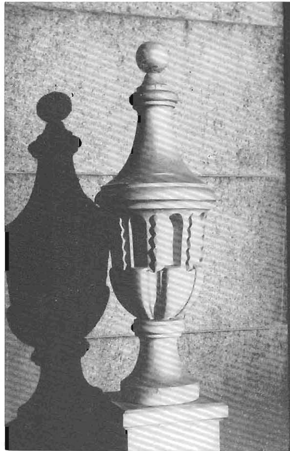
FIG. 11. Original Urn from Roof. One of the seventeen carved wooden urns that ornamented the balustrade on the Library roof has been preserved at the Ridgway Branch. Height, 50½", max. dia. 16½", pedestal modern. Courtesy of National Park Service.
