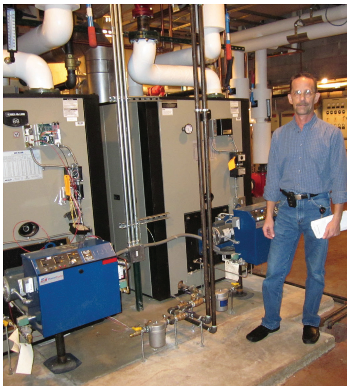
Chief of Maintenance and Security Al Dallasta with the new dual-fuel boilers.
